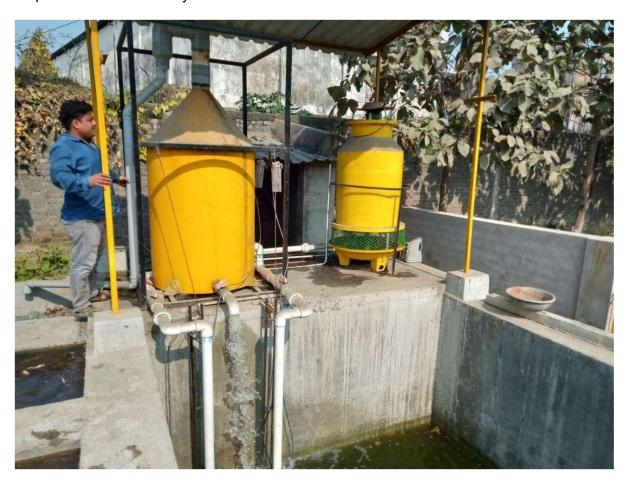
In this stage, further carrying away of **bio growth** with water is prevented. The Nano Bubbles being charged help in coalescence of the impurities and this helps in removal and load reduction by removing them in form of foam. There is no membrane, no maintenance. It is use of aeration for flotation. The resulting water is free of most of the organic load.etc.
