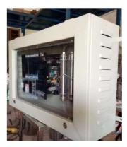
Ozone is injected to kill bacteria in tertiary stage Ozone has a very high oxidation potential. Ozone does not form organochlorine compounds, nor does it remain in the water after treatment. Ozone is a cost-effective method of treating water, since it is produced on demand and does not require transportation and storage of hazardous chemicals. Once it has decayed, it leaves no taste or odour in water.
